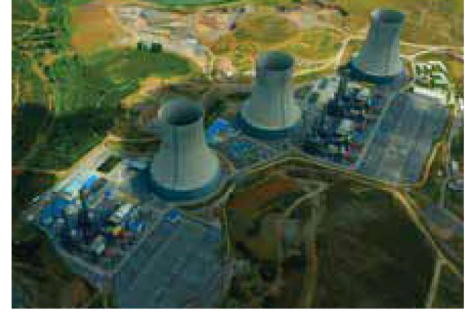
Enka Power Plant – Erbil – Süleymaniye
