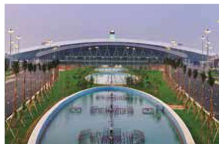
Baiyun International Airport T2 Terminal Guangzhou, China
