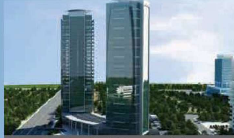
Bayraktar Twin Tower – Ankara
