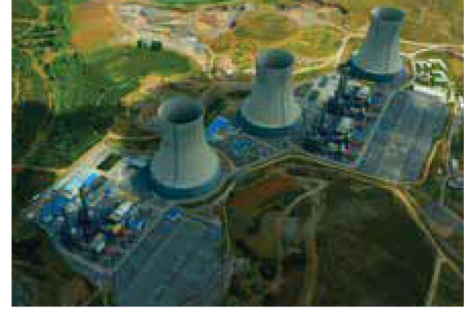
Enka Power Plant – Erbil – Süleymaniye
