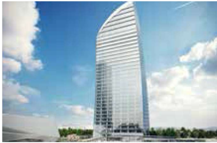
Libeskind Tower Milan, Italy
